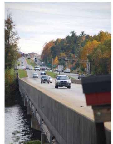
Figure 5.4 – Highway access to the greater region is critically important for Hickory's economic development.
