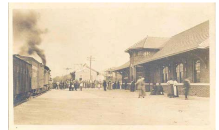
Figure 2.2 – Hickory's train depot, located just south of Union Square.
