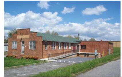
Figure 3.11 – Redevelopment of functionally obsolete industrial buildings is one of the biggest challenges facing the City's rail corridor.
